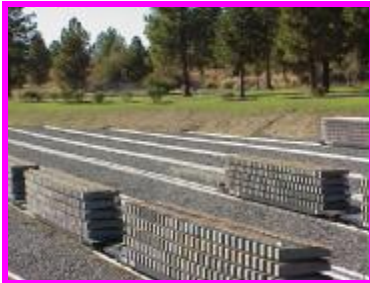
Main Yard Extensions
