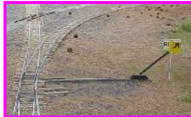
Some main line switches have the 'big throws' on them, the arrow indicates it's direction. These have 'lot's' of leverage, please don't force them!
