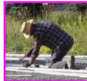
Charlie 'Bill' installing the replacement track in Crisp Yard.
