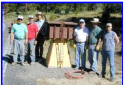
The Water Tower Installation crew
