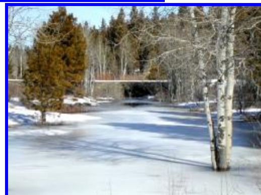
The Train Mountain ice skating rink Dam #1 to Dam #2
