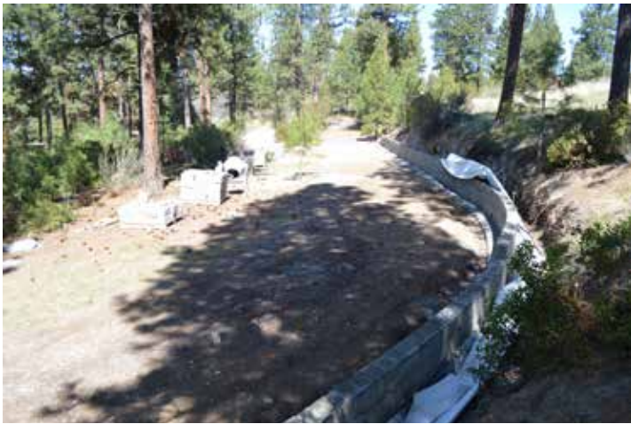
be laid and filled with cement before the Hairpin retaining wall is complete.
