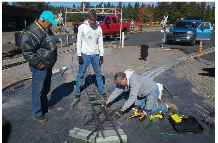
Daniel and Dave Waterstreet install the diamond as Les Dent looks on.
