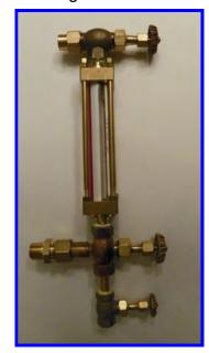
The configuration on the left is incorrect because the Middle Valve will not allow proper blow-down of the Sight Glass. The configuration on the right allows closing the Middle valve, controlling Boiler Water, and opening the bottom valve to drain the Water Level Glass. Steam will exhaust out of the Drain (bottom) Valve.
