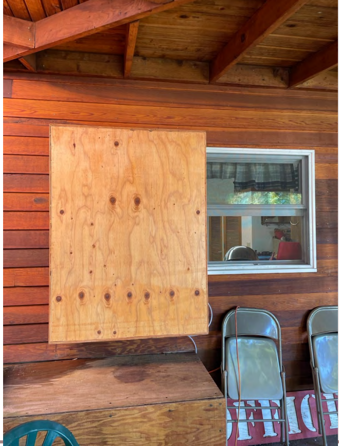
John and Richard Croll built a new winter cover for the kitchen's swamp cooler.
