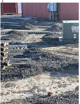
isting meter is expensive. The most economical option is to run a long "extension cord" from the back shop to the meter on the containers and split where we are feeding back into the grid. So that is why the yard is temporarily torn up, and why we are digging a trench!
